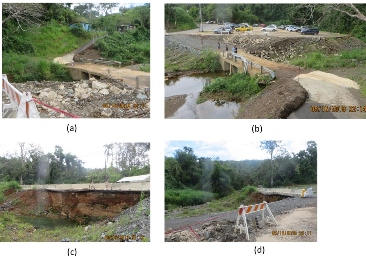
**Figure 4.** A new bridge under construction in Las Marias—heavy flooding resulted in localized landslides and the washout of the original bridge. (a) bridge serving trapped residences, (b) bridge embankment with debris from upstream landslides, (c) scoured embankment, and (d) newly repaired bridge approach. (Photo credit: Shen-En Chen).
