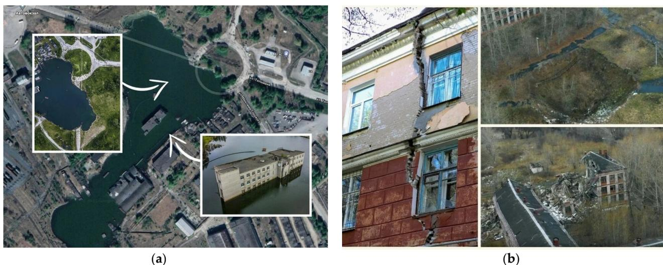
**Figure 5.** Destruction of surfaces and buildings as a result of a man-made disaster in 2006 (Perm region, Russia): (a) sinkhole at the territory of an administrative facility, 2011; (b) sinkhole at the territory of a school, 2015, Berezniki.
