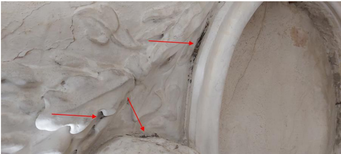
Figure 8. Mold colonies on the stucco of the west wall of the King's Library.
