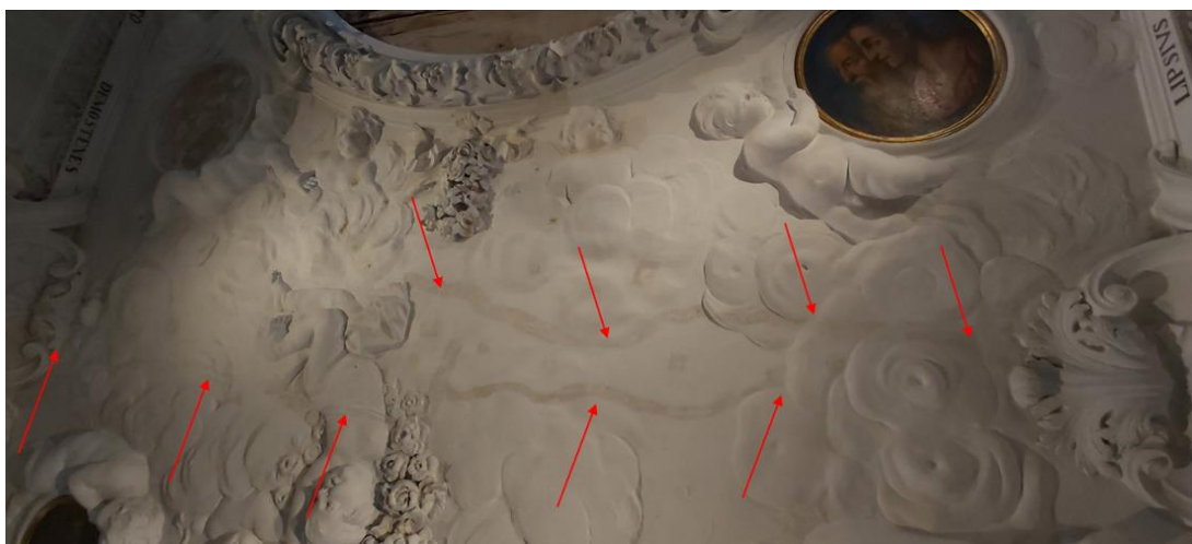
Figure 4. Cracks in the plaster and stucco in the central ceiling of the King's Library.
