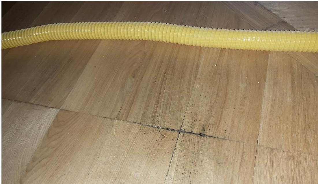
Figure 19. Deformation and discoloration of the oak flooring in the Historical Cabinet, part 1.
