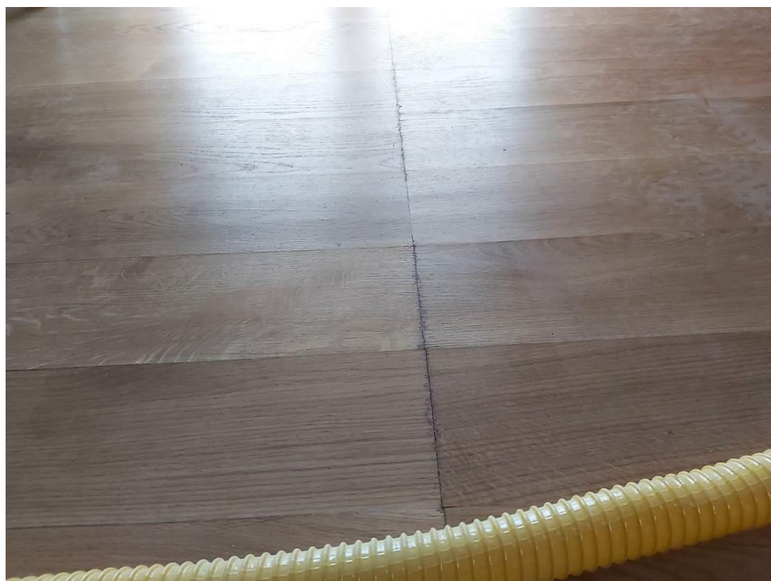
Figure 20. Deformation and discoloration of the oak flooring in the Historical Cabinet, part 2.
