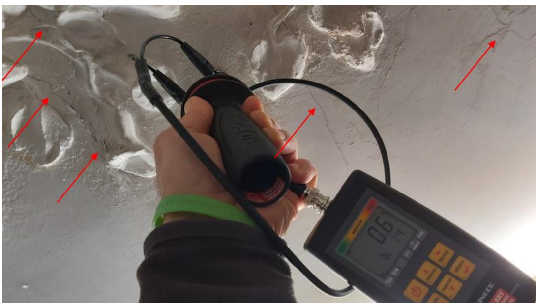
Figure 5. Cracking and chipping of plaster in the southern part of the ceiling of the King's Library.
