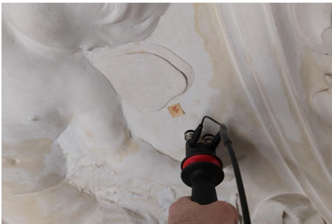
Figure 6. Discoloration of the stucco and plaster on the ceiling of the King's Library.
