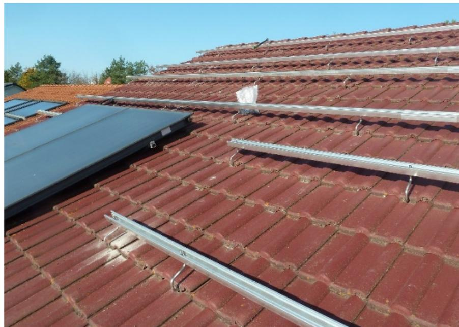
**Figure 1.** Mounting/railing system for a relatively simple 11 kW<sub>p</sub>, residential PV generator on a tiled roof. The roof angle is 25°. Only the two solar thermal collectors on the lefthand side cannot be covered by PV modules. Including wages, the total mounting cost ranged at  $MOUNT_{\square} \approx 40$  EUR/m<sup>2</sup>. Due to the necessary, but time-consuming, process of cutting/adjusting tiles for the roof hooks, this mounting cost is relatively high.
