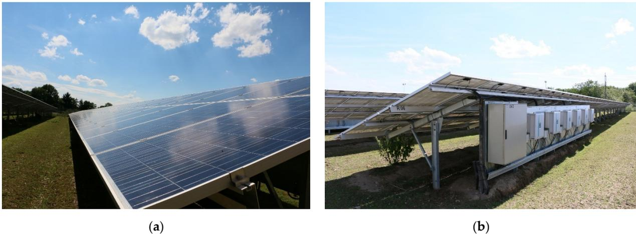
**Figure 3.** A 200 kW<sub>p</sub> PV system mounted in 2013. (a) Front view with multicrystalline Si modules. (b) Back view. The mounting system, contributing to the mounting cost  $MOUNT_{\square}$ , employed in Equation (2), consists of piled steel poles and steel rails. The six inverters and the large box for housing the internet connection are included in the  $FIX_{\square}$  in Equation (2). The total mounting cost was  $MOUNT_{\square} \approx 35$  EUR/m<sup>2</sup>.
