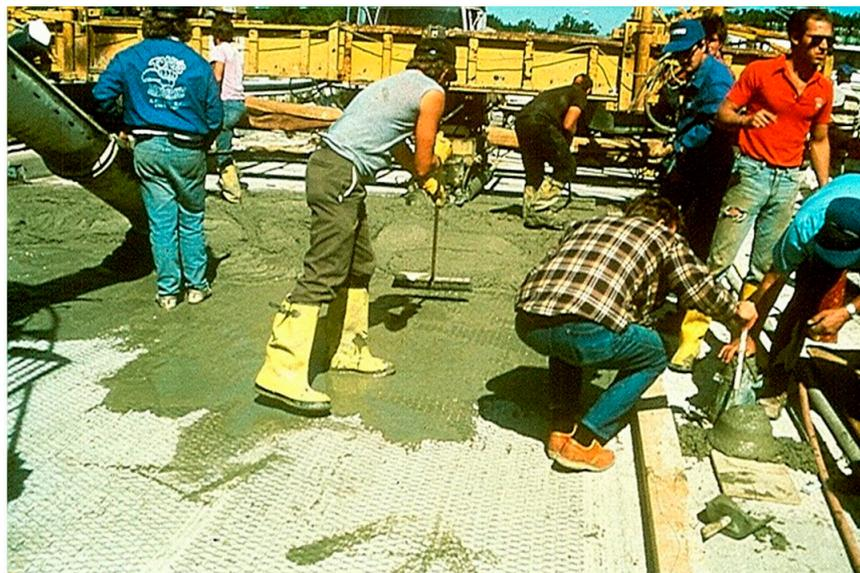
**Figure 3.** Mixed metal oxide coated titanium mesh anode being installed on a ridge deck. Courtesy Jack Bennett. Reprinted from Ref. [1] with permission. Copyright 2007 Taylor and Francis.
