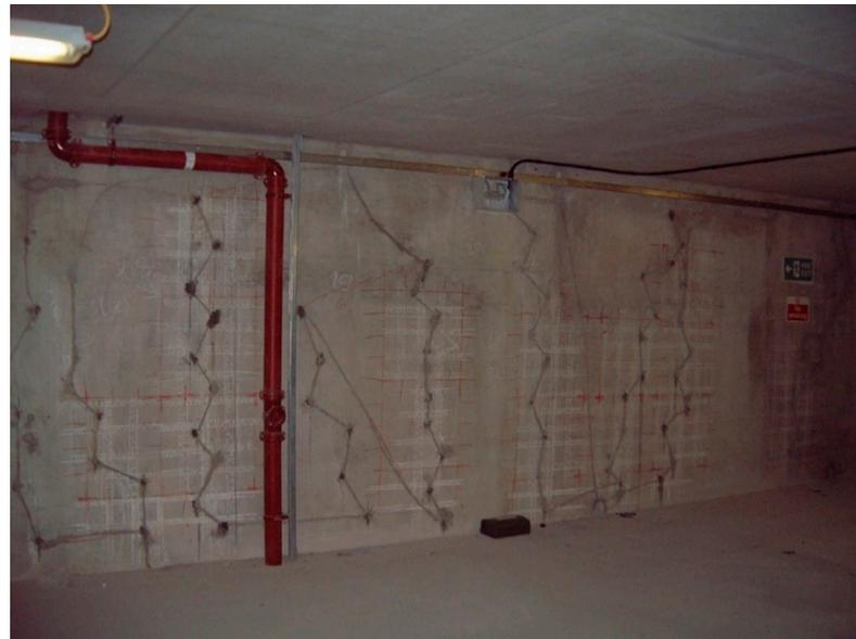
**Figure 5.** Probe anodes being installed in a basement wall to protect the reinforcement where there was chloride ingress and through cracks.
