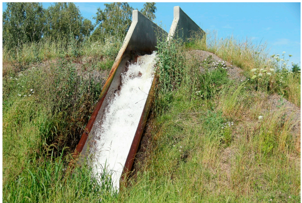
Figure 2. Cascade (staircase) behind the inflow of mine water to the treatment plant.
