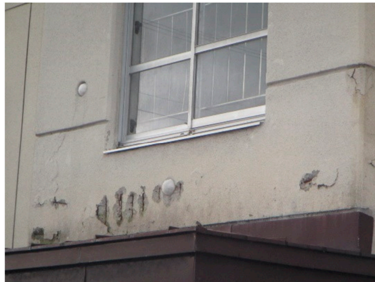
Figure 3. Spalling of concrete due to cracking and corrosion in a cold climate [107].
