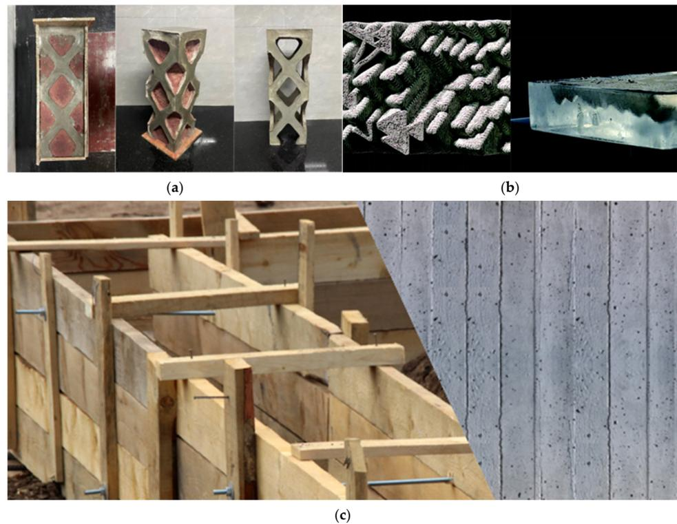
**Figure 1.** Different types of formwork materials. (a) Frozen sand formwork [48]; (b) ice formwork [47]; (c) timber formwork.
