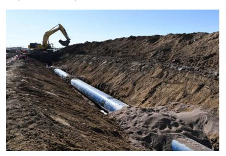
Figure 1. A gas pipeline being buried in construction.
