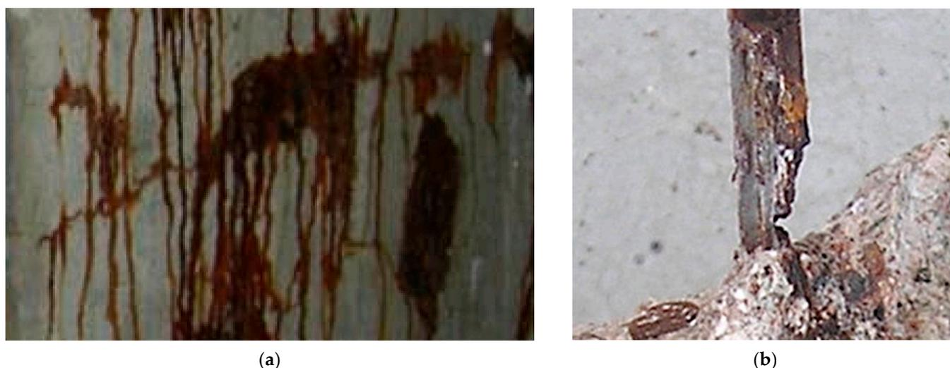
**Figure 9.** Examples of severe localized loss of reinforcement steel from (a) corrosion inside through wall cracking of 40-year-old Sydney Harbour ammunition lighters showing the typical red-brown corrosion stains left by oxidation of ferrous chloride and (b) example of highly localized corrosion of reinforcement steel (6 mm dia.) at a location coinciding with a crack from the external wet saline environment.
