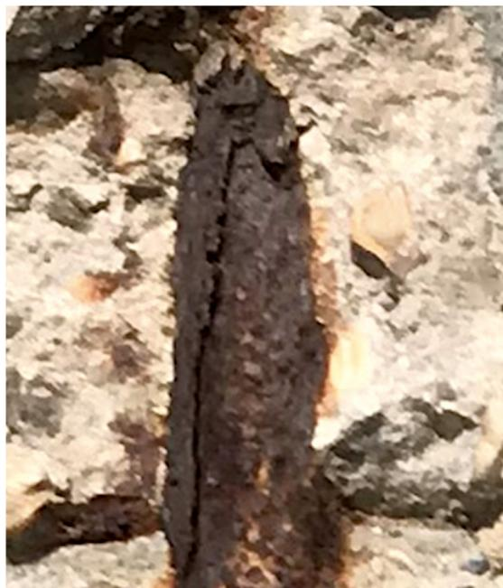
**Figure 10.** Close-up view of exposed reinforcement bar showing corrosion on the outer surface of the bar but negligible corrosion at the sides and negligible corrosion products into the concrete surrounding the bar (detailed view of bar in Figure 4b).
