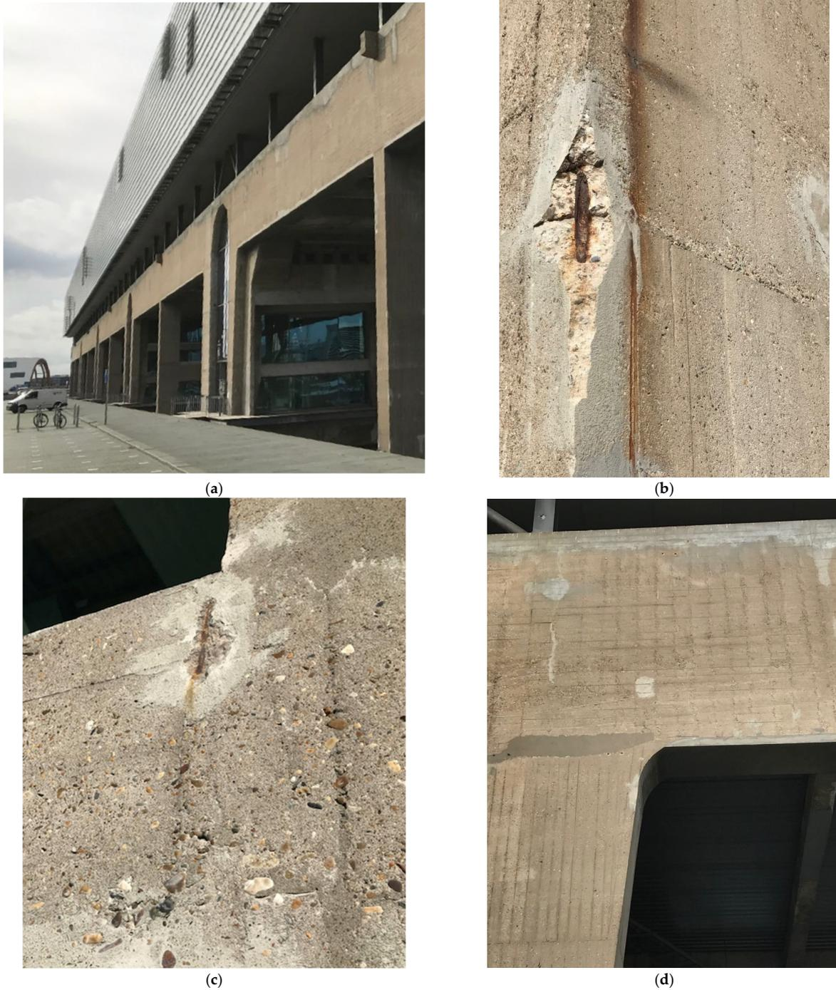
**Figure 4.** (a) Overview of 1950s Kraanspoor reinforced concrete structure with recently constructed superstructure (b,c) localised loss of concrete cover and reinforcement corrosion at corners of portal frame columns in 2019, showing some evidence of (unsuccessful) patch repair, (c,d) examples of flat off-form concrete surface showing alignment of the reinforcing bars underneath.
