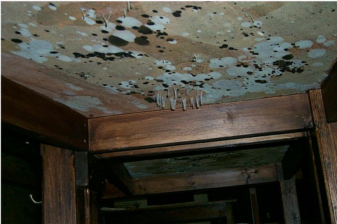
Figure 6. Mould on the underside of plotting table in Gun Operations in 2002.
