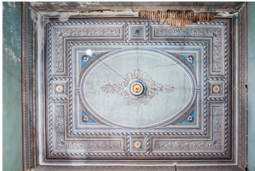
Figure 19. Ceiling paintings in the dining-room, where the bagdati construction is visible. Photograph by Panagiotis Ilias ©.
