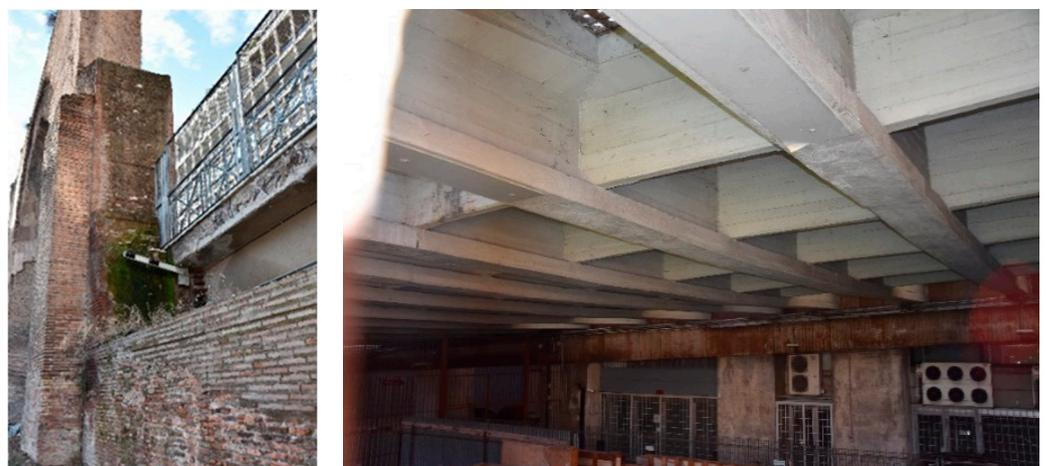
**Figure 13.** The fragmented wall of the gymnasium and the reinforced concrete slab supporting Via Parigi.
