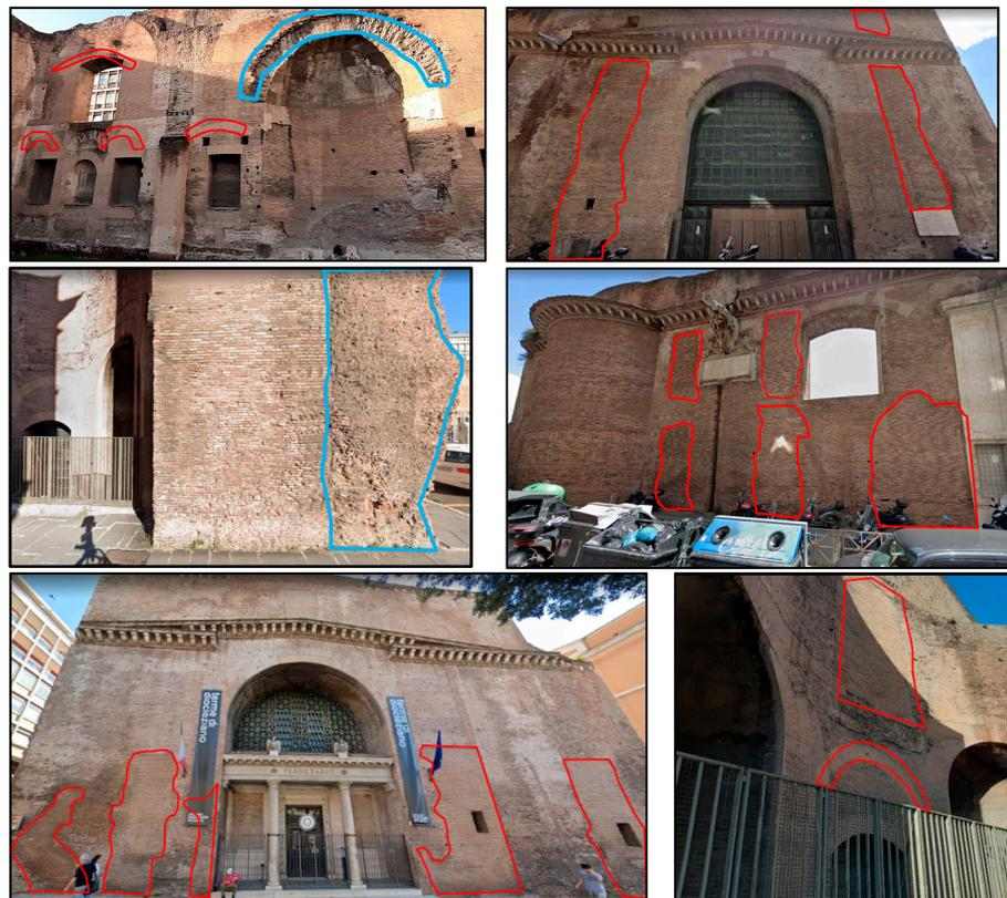
**Figure 6.** The main damaged parts (highlighted in blue) and the visible restorations (highlighted in red).
