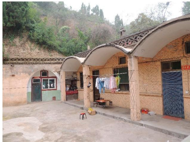
**Figure 4.** Underground village around the Wang Family Compound in Shanxi Province (China). New cave dwellings have been built in yaodong style annexed to the traditional ones that have been partially abandoned or adapted to the needs of modern life (by F.F. and L.L., 2017).
