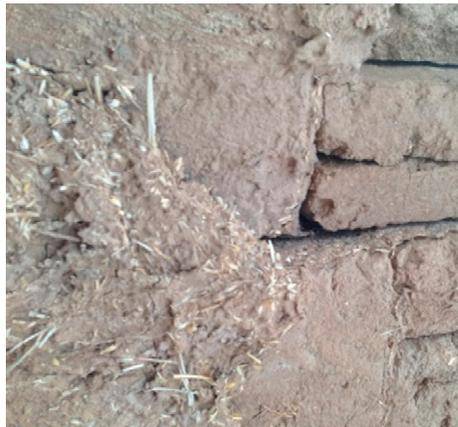
**Figure 7.** Lijiashan Village in Shanxi Province (China). Mud bricks made of the earth of Loess (by F.F. and L.L., 2017).
