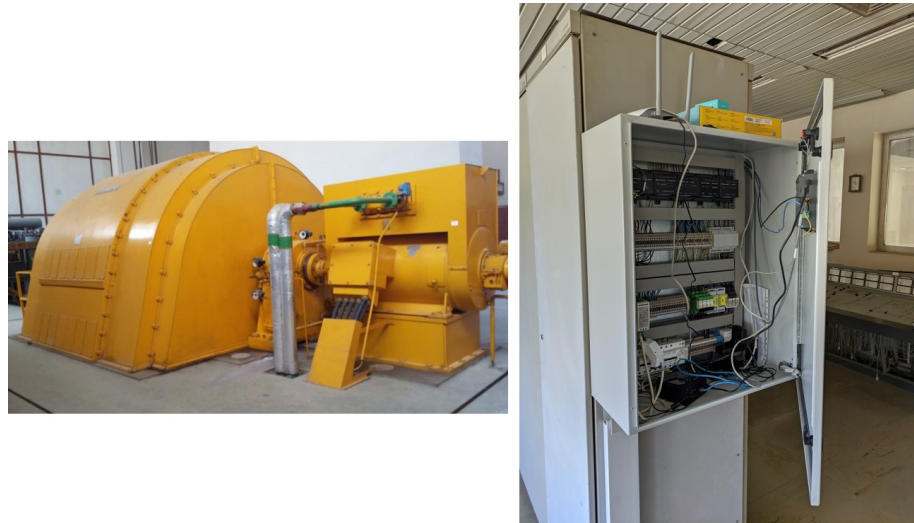
Figure 3. Power generator (left) and RTU integration within PPC infrastructure (right).
