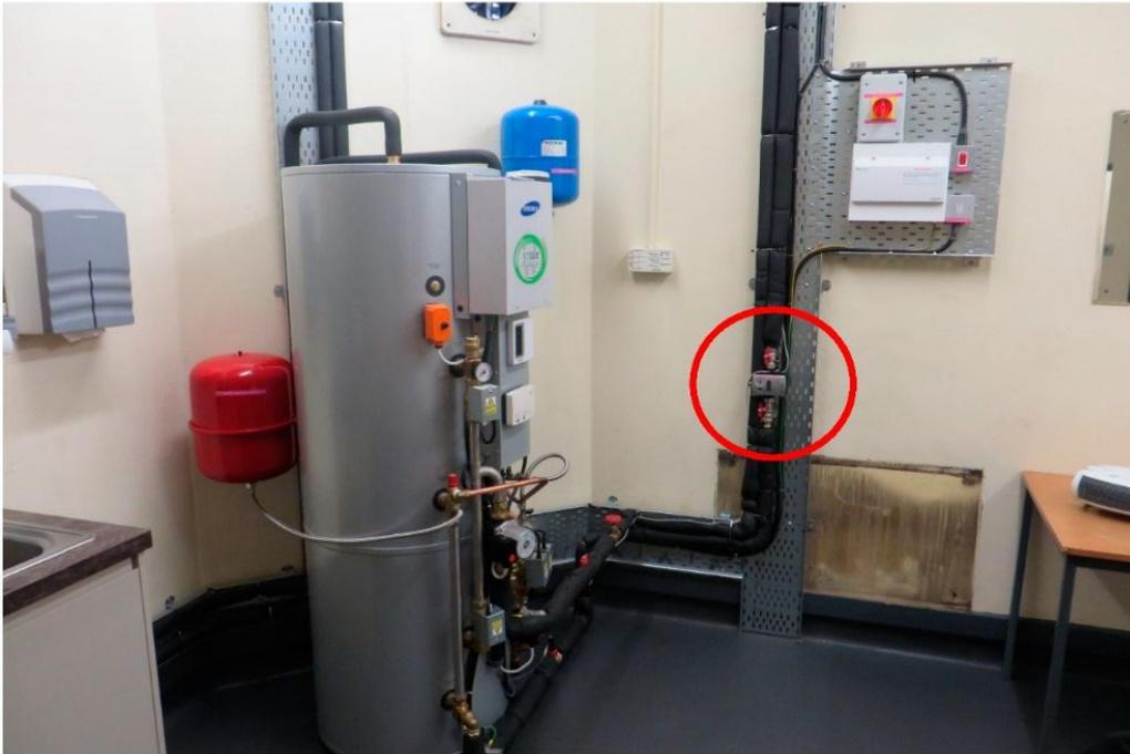
**Figure 4.** The compact indoor unit of the heat pump and the energy meter (in red circle).
