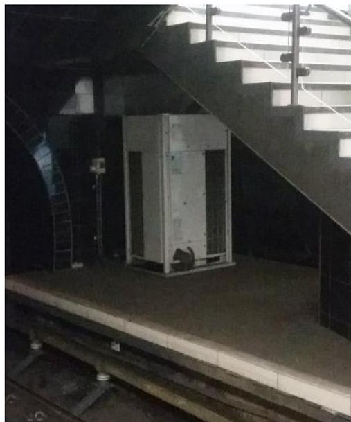
**Figure 10.** Buchanan Street Station's ASHP below the stairs at platform level.
