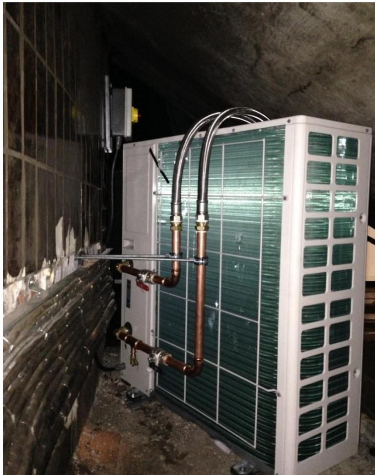
Figure 7. The condenser under the stairs at platform level, positioned on an angle.
