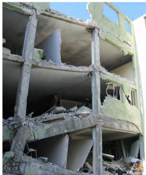
Figure 1. Lean-to-collapse pattern in reinforced concrete building [14].
