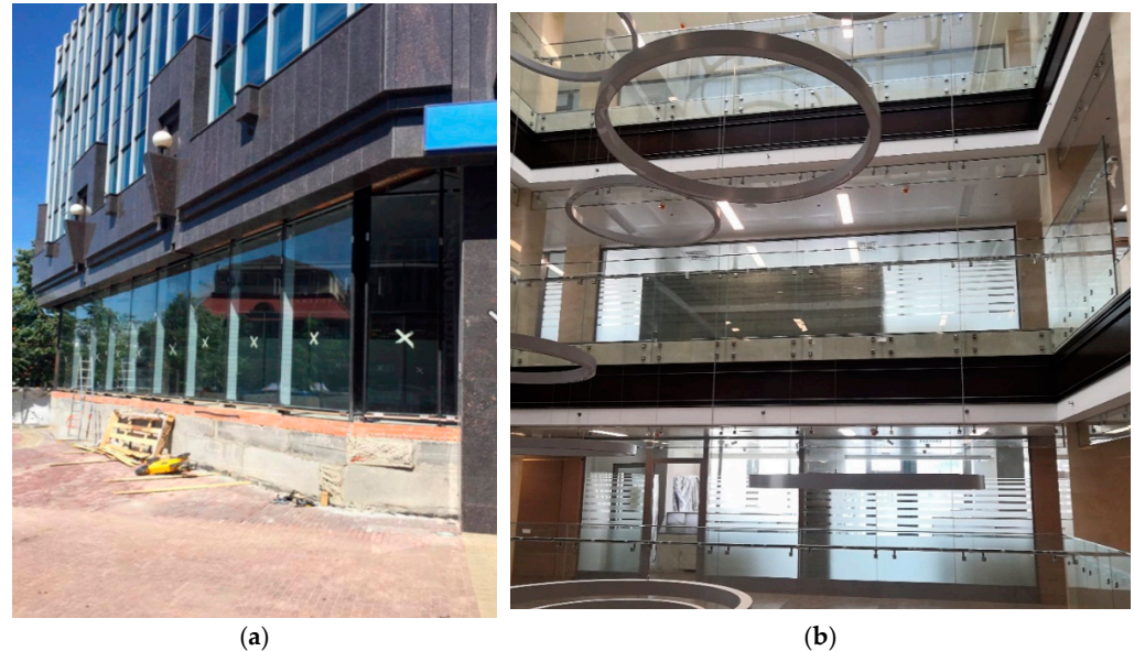
Figure 1. Business center “Chelyabinsk City”: (a) facade and (b) smoke-proof all-glass screen in the atrium. Photo by the authors.
