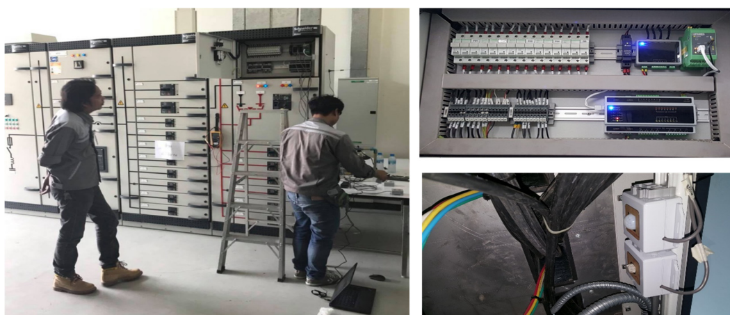
Figure 3. A display of an intranet sensors system installment in various electrical switchboard settings.
