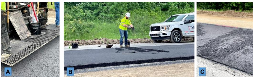
**Figure 2.** MTM 324 inspection for I-69 project (A: Sampling plates and wires, B: Taking samples, C: Filling the voids).
