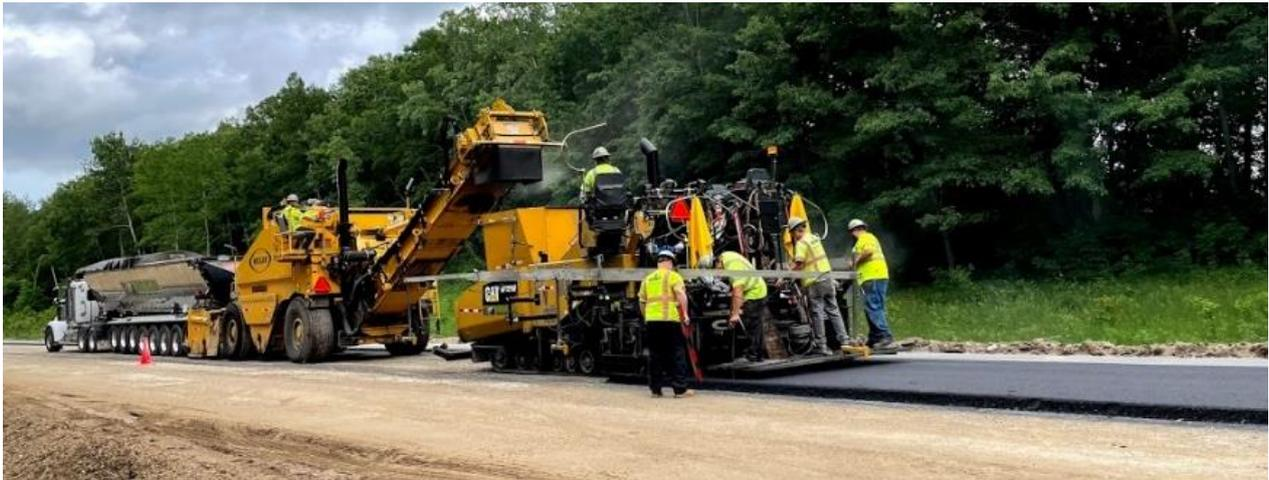
**Figure 8.** I-69 HMA pavement construction operation.
