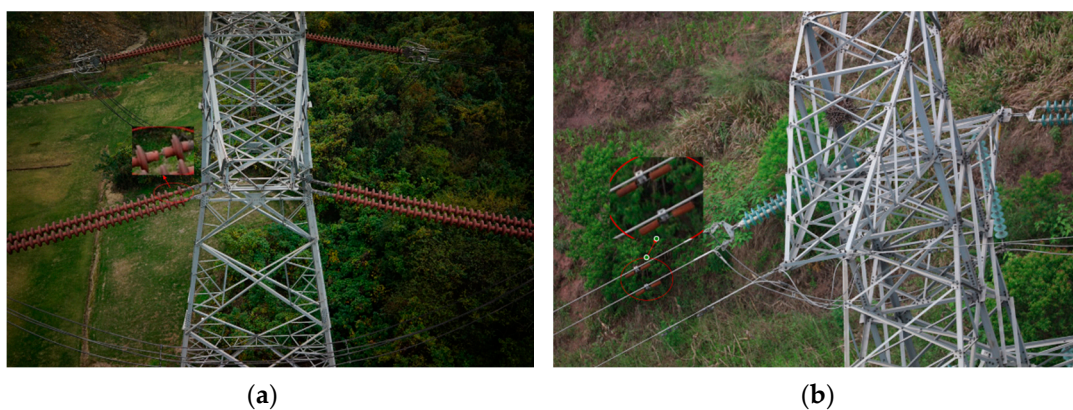
Figure 10. (a) Example of a broken insulator in a small target; (b) example of vibration hammer rust in small targets.
