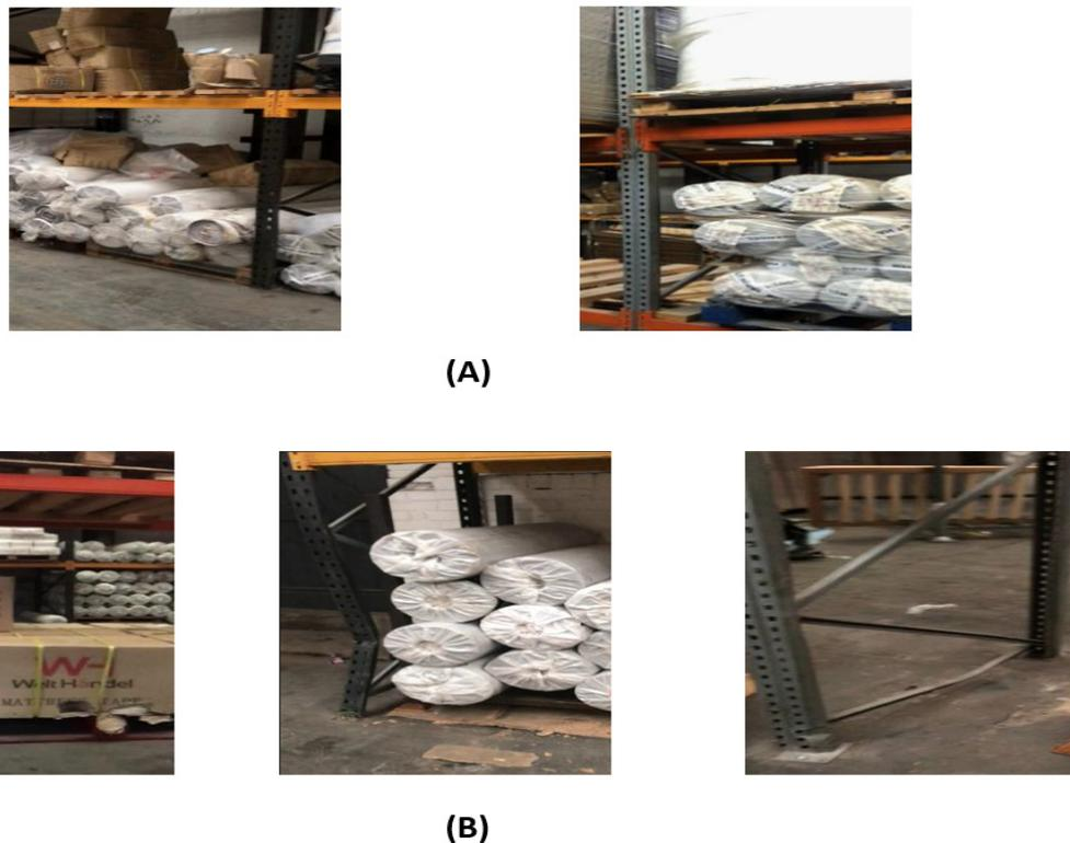
**Figure 1.** Original dataset. (A) Normal and (B) damaged racking.
