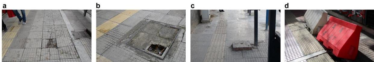
**Figure 5.** Examples (a–d) of uneven and dangerous parts of sidewalks with poor cleanliness and obstacles hindering walkability and increasing the risk of falling or tipping.
