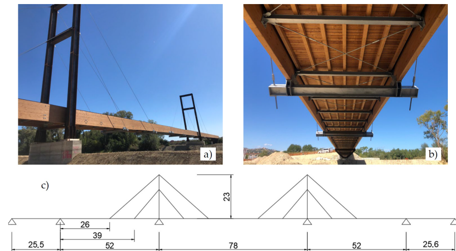
Figure 2. Footbridge case study: (a) lateral view, (b) bottom view, (c) geometric scheme (measured in meters).
