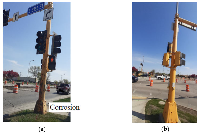
Figure 1. Images of existing traffic poles (a) exhibiting significant corrosion; (b) without major corrosion.
