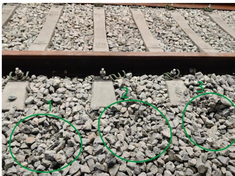
**Figure 4.** Holes dug in the ballast (marked in green).
