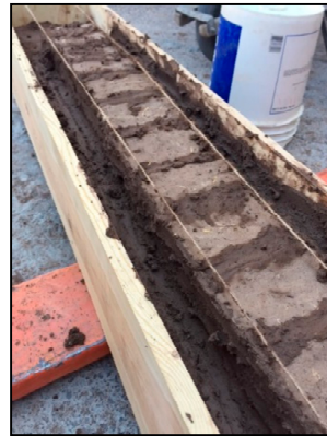
Figure 1. Construction of the wall foundation: Adobe bricks being placed in the wooden frame to form the footing.
