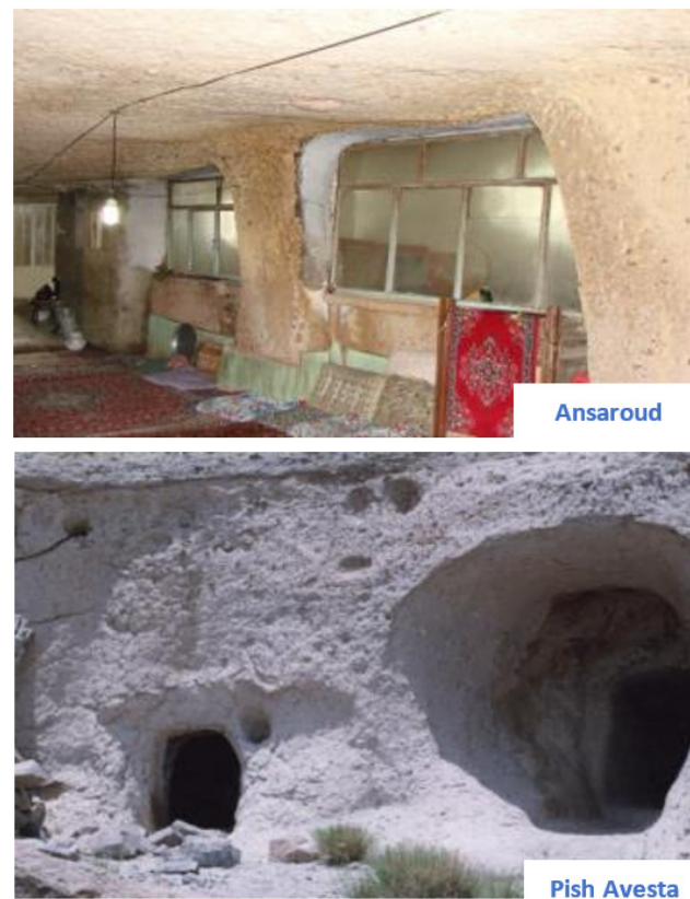
Figure 15. Difference in the size of the particles led to difference in the quality of excavation in Ansaroud Grand Mosque and Pish Avesta Temple.
