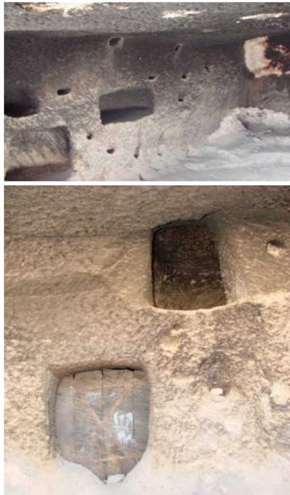
Figure 13. Fine excavation technique used in doorways, niches and interior space of rock-cut rooms in Meymand.
