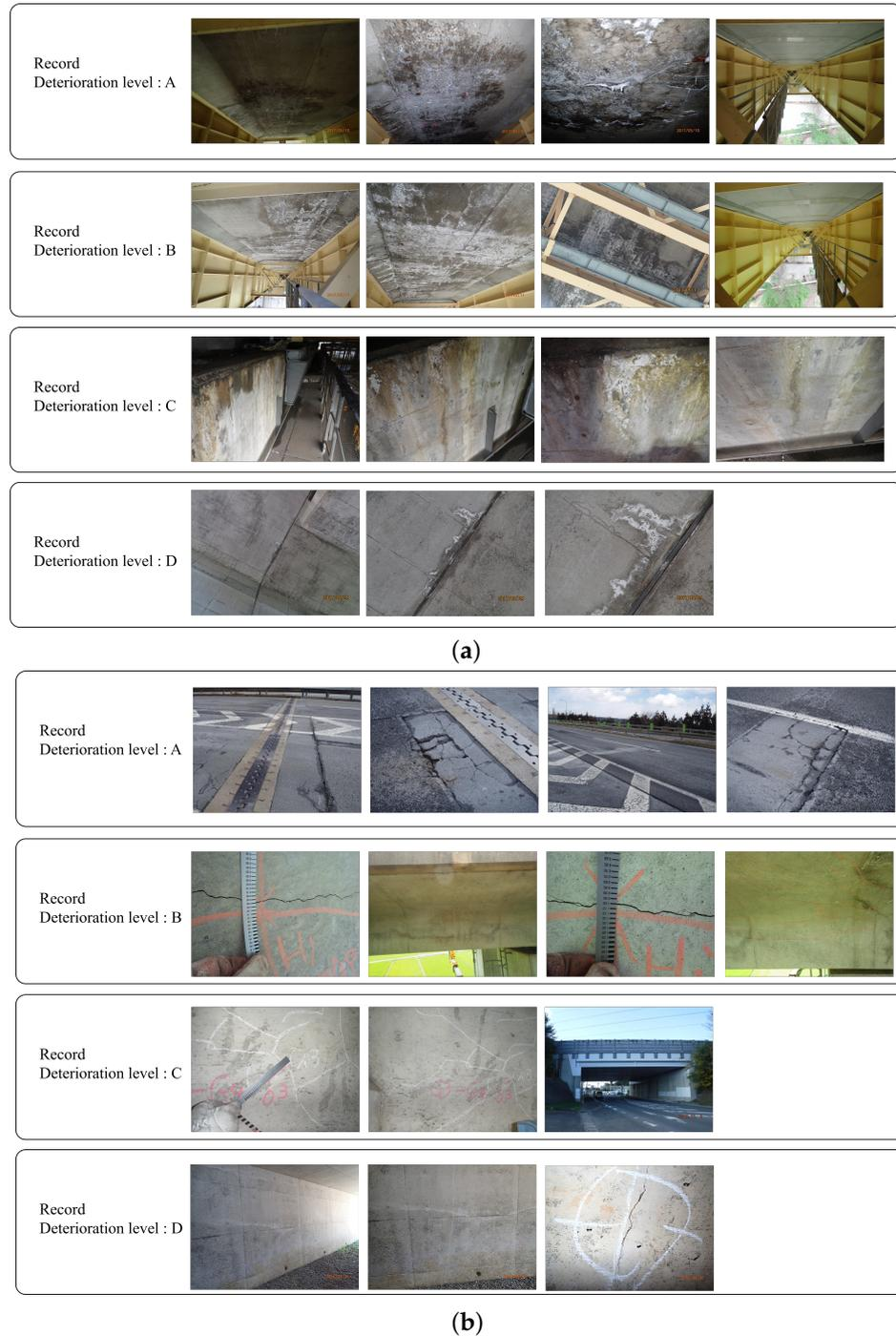
**Figure 4.** The examples of distress images in records. (a) Efflorescence and (b) Crack.
