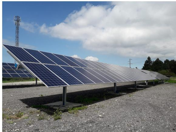
**Figure 1.** Solar PV panel equipped with a single-axis torsional system to rotate and maximise the incidence angle. Image provided by Gonvarri Solar Steel.
