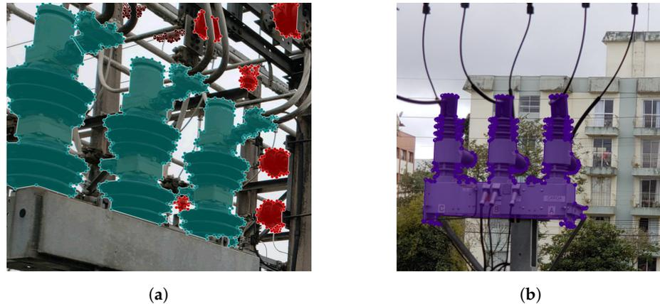
**Figure 6.** Examples of manual annotation for semantic segmentation using LabelMe. The colors used by LabelMe have no relation to the colors used in the masks from Table 3. (a) Insulators (red) and breakers (green). (b) A recloser (purple).
