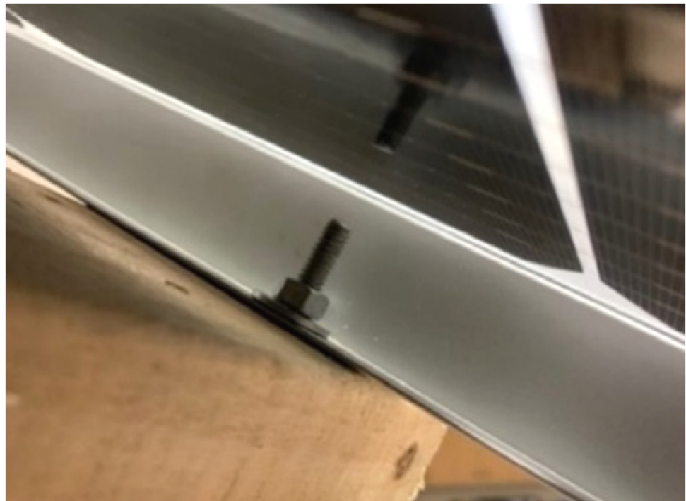
Figure 7. Simple standard steel bolts can be used to attach a conventional PV module to a wood frame. The reflection of the bolt is seen in the PV cell in the bifacial module above it.
