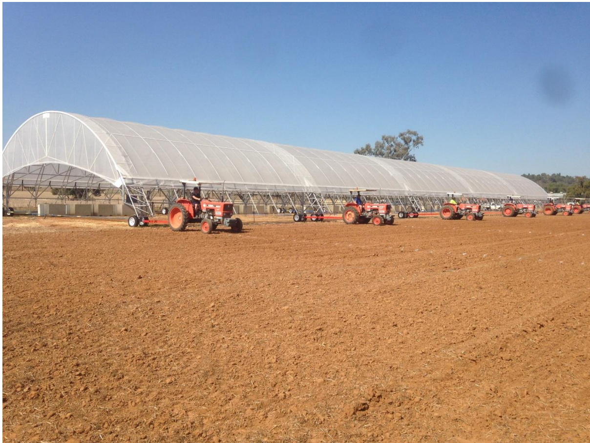
Supplementary Figure S1: Layout and movement of rainout shelter at the Wagga Wagga Agricultural Institute, NSW Department of Primary Industries, Wagga Wagga, Australia. Five rainout shelters (ROS, each was 15 m length x 15 m wide) were designed and built by Southern Irrigation Pty Ltd (Leeton, NSW, Australia). Each rainout shelter was covered with a polyethylene sheet (Polytex, Leeton, NSW, Australia) and then joined end to end. Junctions were covered with a polyethylene sheet, as shown. An array of five ROS (15 m long x 75 m wide) was hooked via a hitch with six tractors and moved to the prepared experimental site (as shown above). This 'polytunnel' was used for experimentation. Heavy-duty metal drainage ensured proper water deficit treatments. In addition, rainwater is directed away from research plots by resurfacing the area surrounding the ROS. Shelters were supported by concrete blocks (~1 ton) and the wheels locked into place to protect from strong winds. Orientation was north-south. Water-deficit block was located towards the north.
