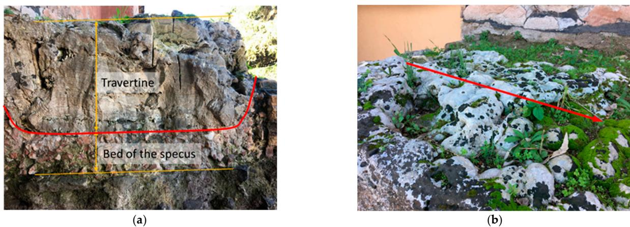
**Figure 16.** (a) A view of the *Anio Novus* aqueduct's travertine deposits on the specus. (b) View from the top of the travertine deposits and their roughness.
