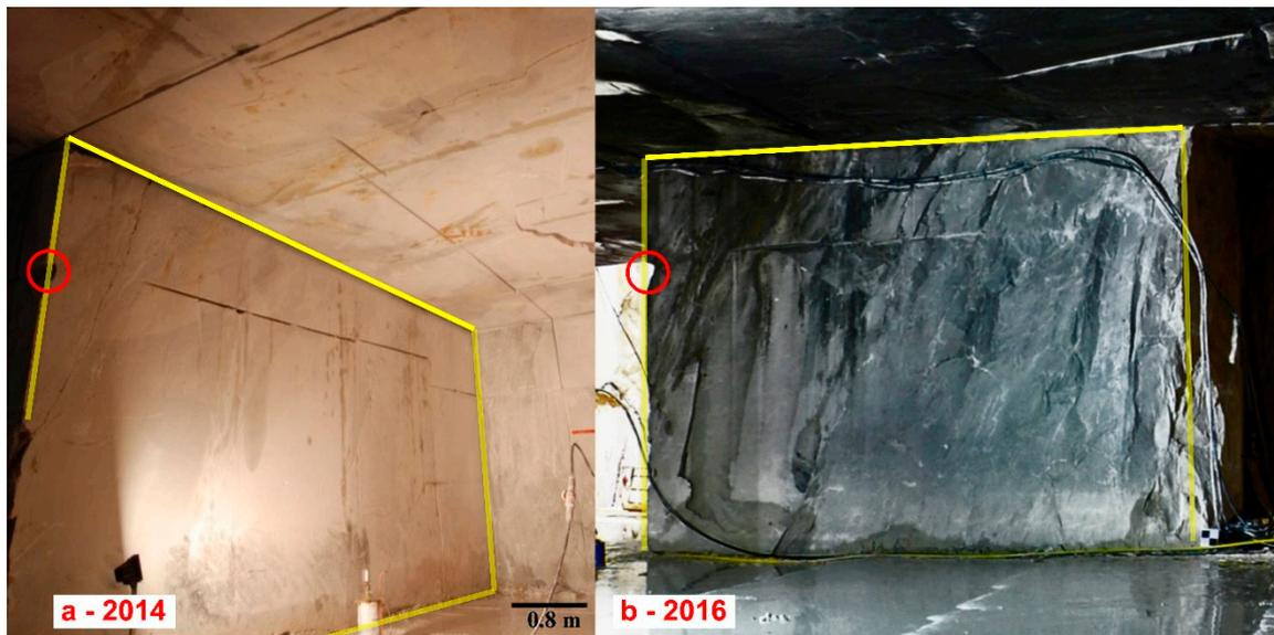
**Figure 1.** Pillar structural condition in 2014 (a)—regular rocky surface after excavation) and 2016 (b)—rough rocky surface after spalling). The yellow box represents the same cutting surface. A common point between the images is highlighted by a red circle. Due to the prospective view, the scale bar is indicative only.
