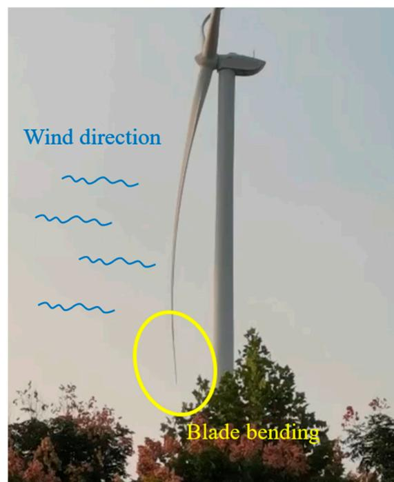
**Figure 1.** Wind turbine blade bending.
