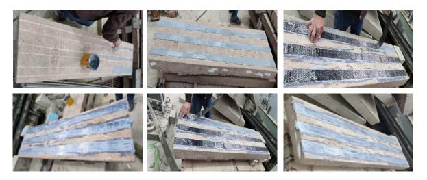
Figure 11. CFRP sheet installation.
