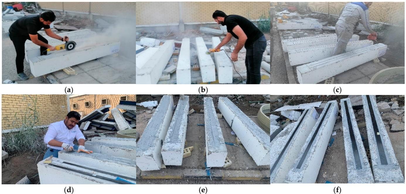
**Figure 2.** Surface preparation and CFRP installation of the RC beams. (a) Making the grooves for NSM group. (b) Surface cleaning and roughing for EBR group. (c) Cleaning the beams from dust. (d) Strengthening the beams with epoxy adhesive. (e) NSM group after strengthening. (f) EBR group after strengthening.
