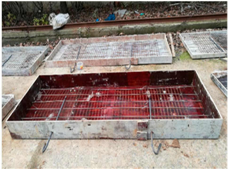
Figure 4. Mold making and steel binding.
