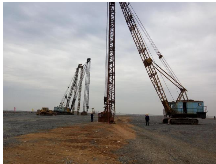
(a) The hauling-up device for dynamic compaction.
