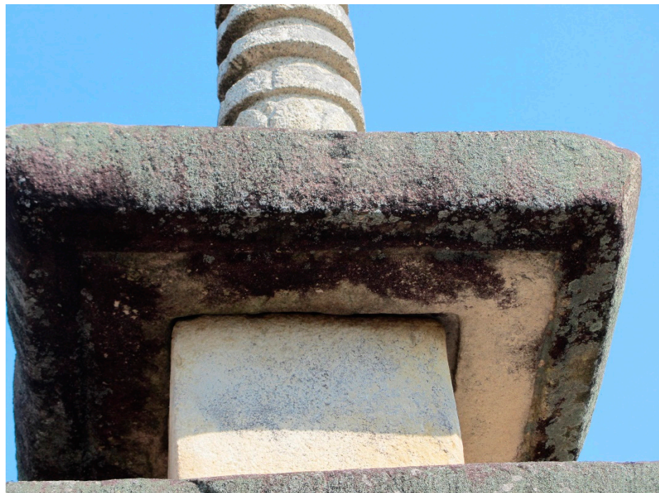
Figure 2. The groove below the eaves at the top story of the Ishidōji pagoda.
