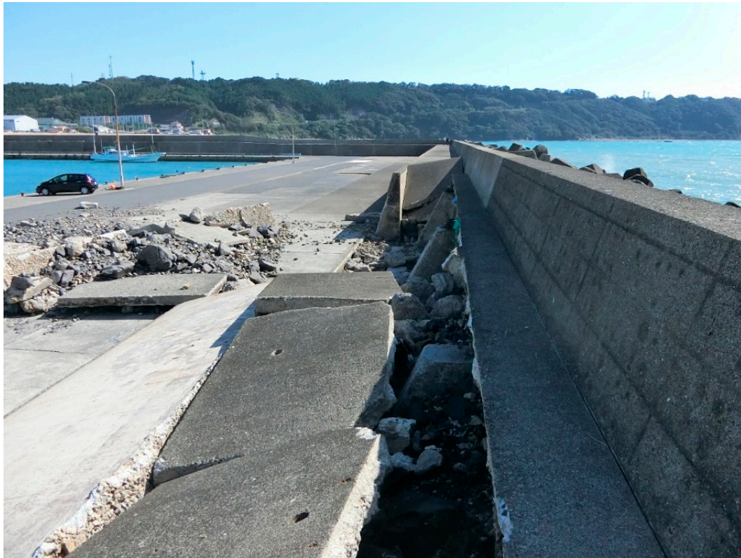
Figure 4. Photograph showing the damaged breakwater observed at Suganohama fishery harbor in Kushimoto, taken by the authors on 2 October 2018.
