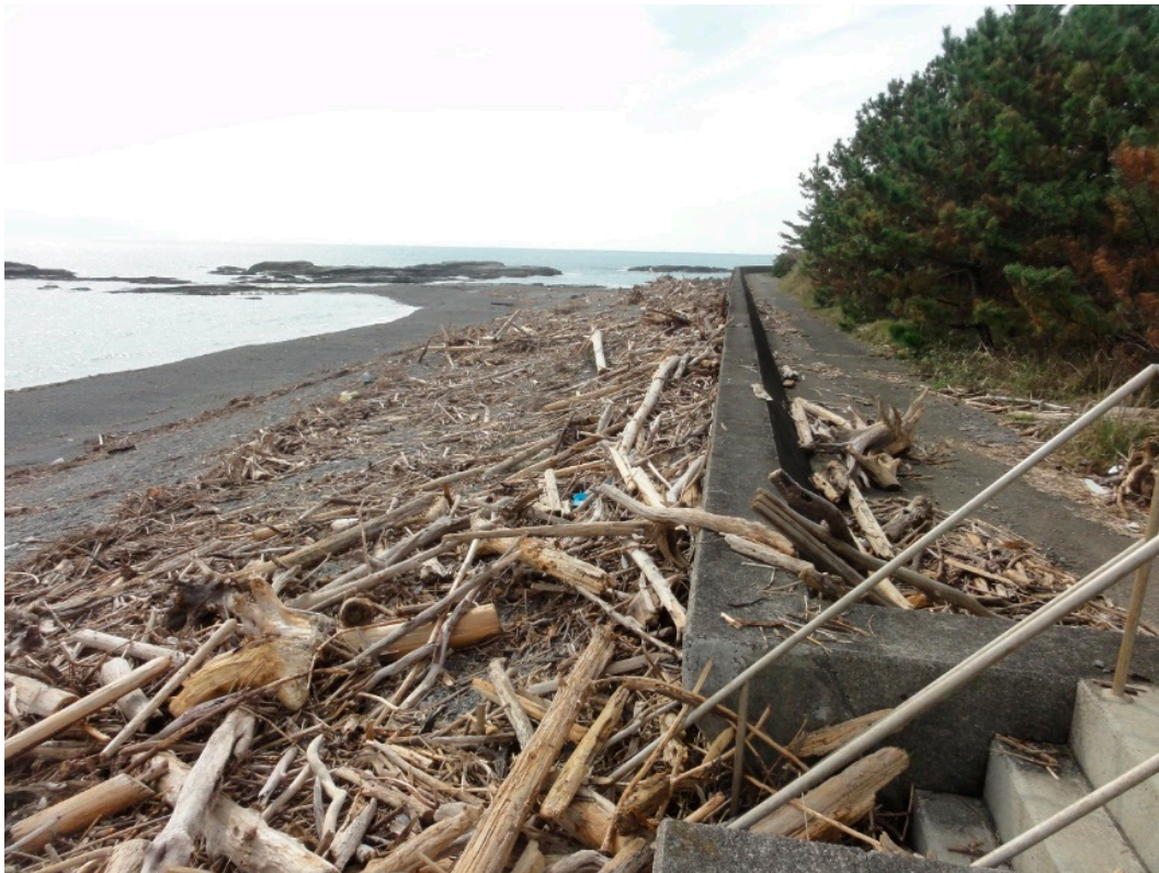
Figure 2. Photograph of debris observed on Tonda Beach with a seawall having a crown height of + 9.2 m from the mean sea level near the head of Tokyo Bay (i.e., Tokyo Peil, TP), taken by the authors on September 21, 2018.
