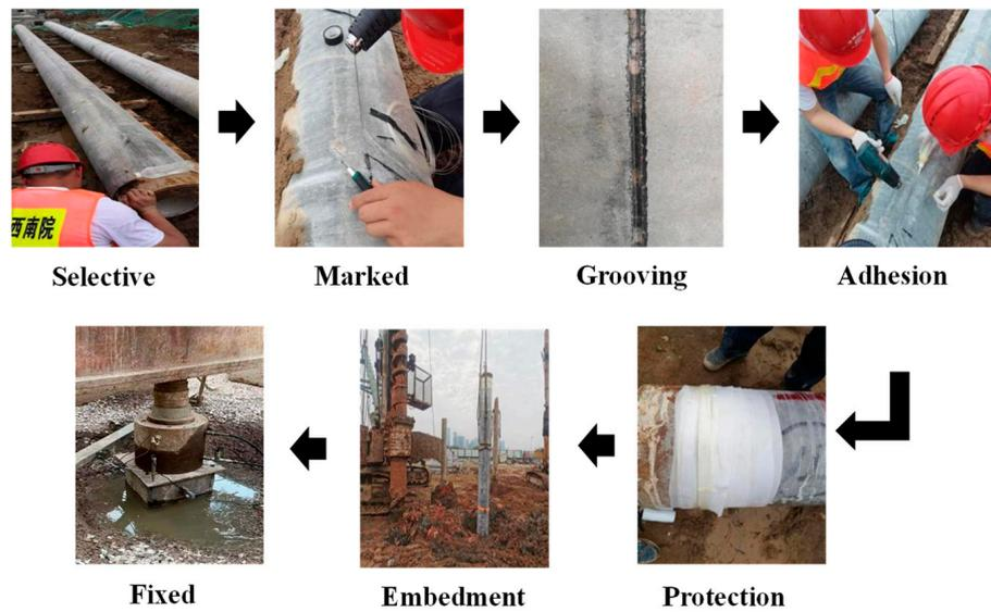
Figure 2. Single pile test layout procedure.
