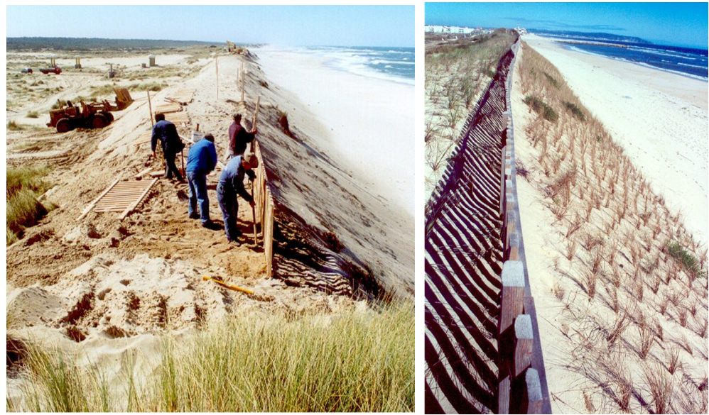
Figure 11. Leirosa sand dune system: artificial reconstruction of the sand dunes followed by re-vegetation with Ammophila arenaria [70].
