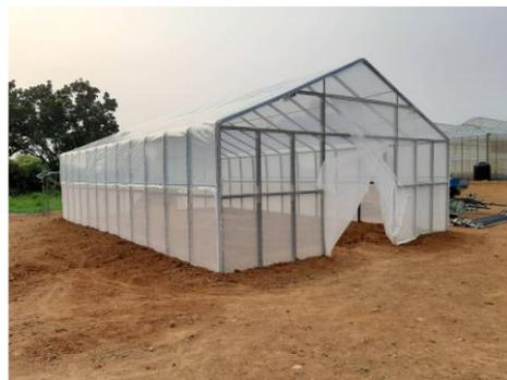
**Figure 7.** The completed structural frame and glazing bars.
