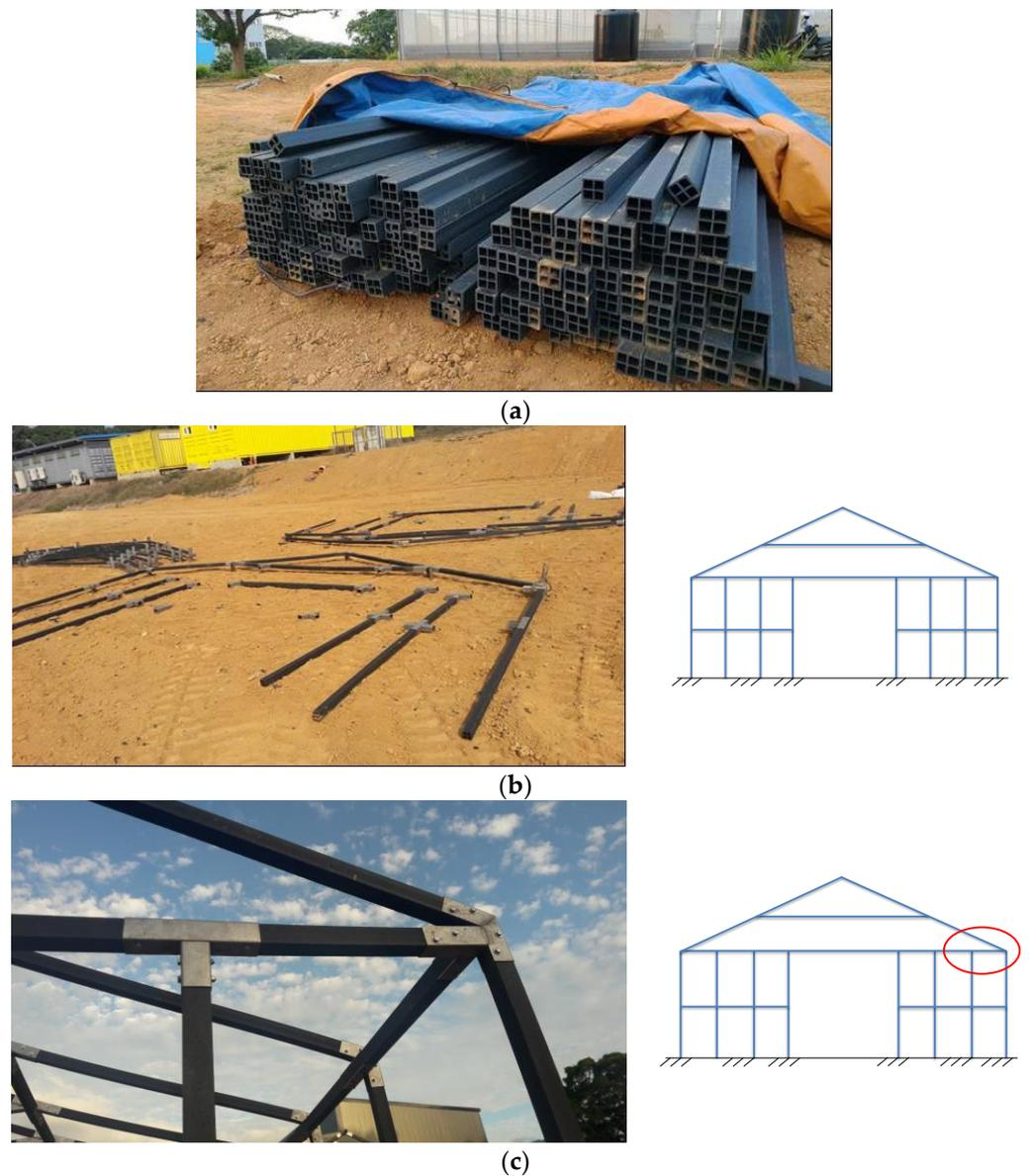
**Figure 5.** (a). Raw members delivered from the manufacturer. (b). Assembling process of the gable frames. (c). Joint fastener of the column, rafter, and joist.
