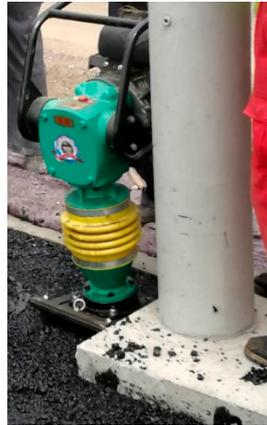
**Figure 5.** The compaction by the plate tamper near the structural edge.
