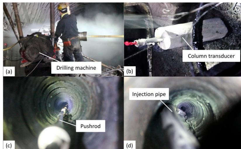
**Figure 10.** Test process for the RSR method in the PDS No. 1 coal mine: (a) Drilling the hole; (b) installing the column transducer; (c) connecting the pushrods; (d) injection pipe for grouting with the cement mortar.
