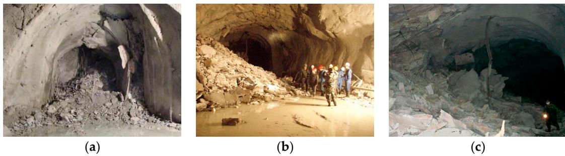
**Figure 2.** Rockburst in auxiliary tunnels: (a) Extremely strong rockburst; (b) induced collapse and (c) support structure damage.
