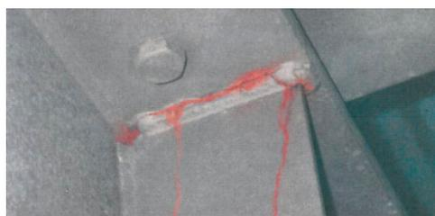
**Figure 1.** Typical fatigue crack in uncoated weathering steel bridges.
